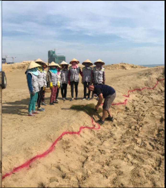
Shaper Matt marking Bunker Edge - September 20
